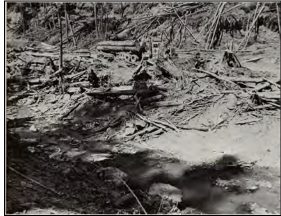
Figure 1-6. Typical 1960s Stream Crossing Through Mainstem Big Salmon Creek, Possibly Located Near Elliot Road (SFPWM 1965-66).
