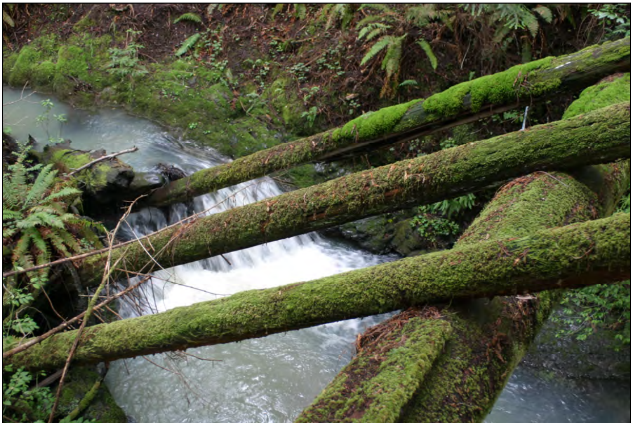
Figure 1-2. Remnant Dam Structure on Hazel Gulch
