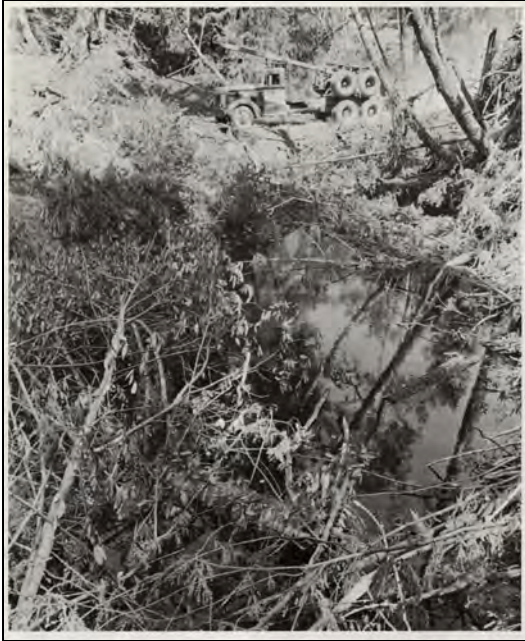
Figure 1-4. Typical 1960s Era Stream Crossing, Possibly Located in Donnelly Gulch (SFPWM 1965-66).
