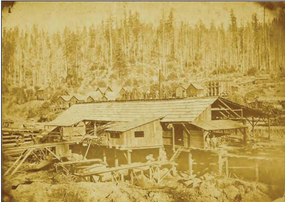
Pullen Mill on Salmon Creek in Albion (photo courtesy of the Mendocino County Historical Society, date unknown)
