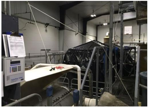
Figure 4. Properly opened and secured drum filter cover
