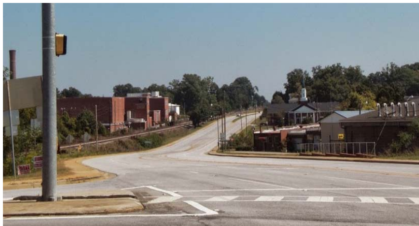
Pedestrian crossing at the intersection of SC Highway 81 and SC Highway 72.
