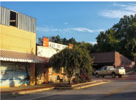
Sidewalk improvements in downtown Calhoun Falls.
