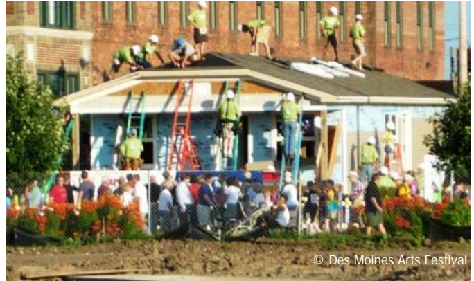
Community Arts Blitz Build for Habitat for Humanity
