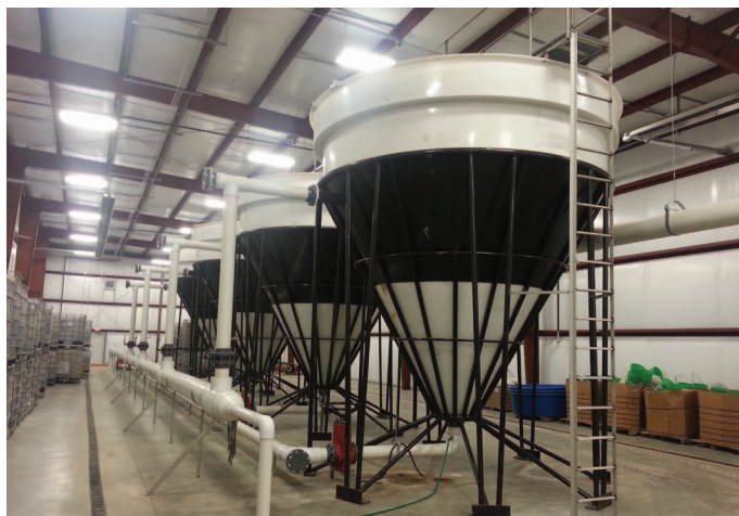
LEFT, FIGURE 3. Submerged filters (left), moving bed biofilters (middle) and trickling filters (right) in the central water treatment area at Langsand Laks, Denmark (Photo: Steven Summerfelt/The Conservation Fund). RIGHT, FIGURE 4. Bell Aquaculture LLC (Albany, Indiana, USA) uses four gravity thickening settling units (each 4 m dia x 5.5 m deep) to capture and dewater biosolids in their RAS facility discharge before this flow is further treated in a created wetland (Photo copyright © 2014 Bell Aquaculture LLC™ — All Rights Reserved).
