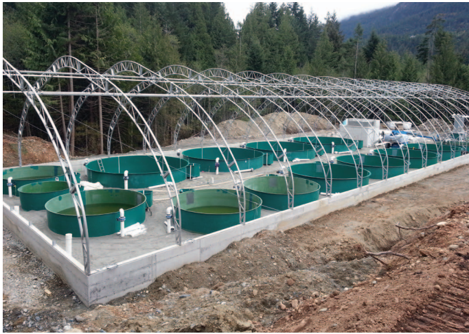
LEFT, FIGURE 1. Hoop building installation in April 2013 at the 100 mt land-based steelhead model aquafarm at Taste of BC in Nanaimo, British Columbia (Photo: Steven Summerfelt/The Conservation Fund). RIGHT, FIGURE 2. The 'Namgis First Nation's "Kuterra" land-based salmon farm uses five 500-m 3 dual-drain culture grow-out tanks connecting to a central water treatment system (Photo: J.R. Rardon).
