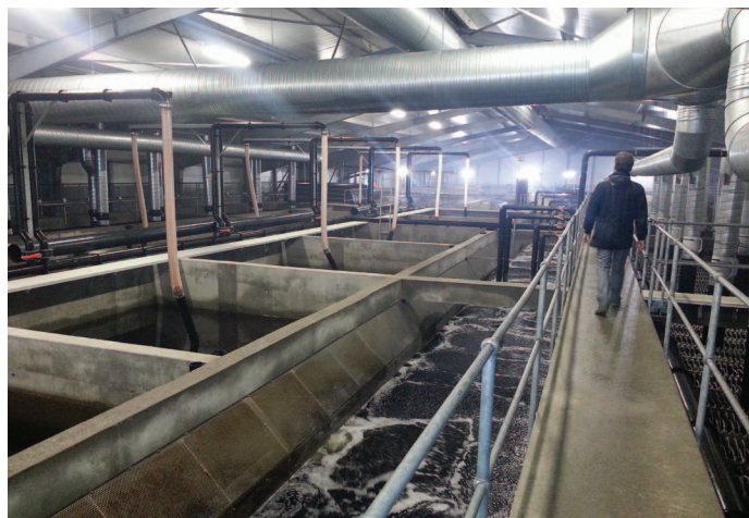
LEFT, FIGURE 3. Submerged filters (left), moving bed biofilters (middle) and trickling filters (right) in the central water treatment area at Langsand Laks, Denmark (Photo: Steven Summerfelt/The Conservation Fund). RIGHT, FIGURE 4. Bell Aquaculture LLC (Albany, Indiana, USA) uses four gravity thickening settling units (each 4 m dia x 5.5 m deep) to capture and dewater biosolids in their RAS facility discharge before this flow is further treated in a created wetland (Photo copyright © 2014 Bell Aquaculture LLC™ — All Rights Reserved).
