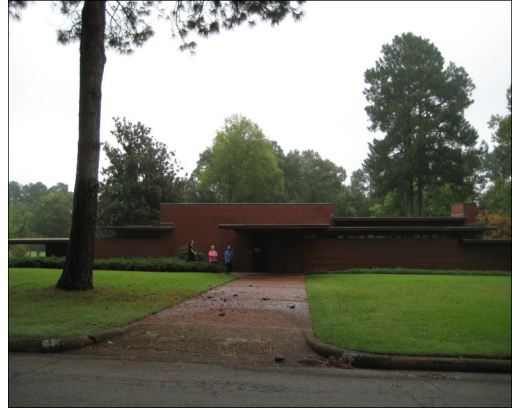
Visitors come from all over the country to see the home designed by famed architect Frank Lloyd Wright. Photo by Carolyn Brackett
