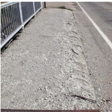
West Portal Road Bridge
