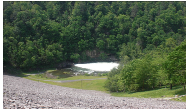
Flannagan Dam Spillway Photo by Kendra Briechle
