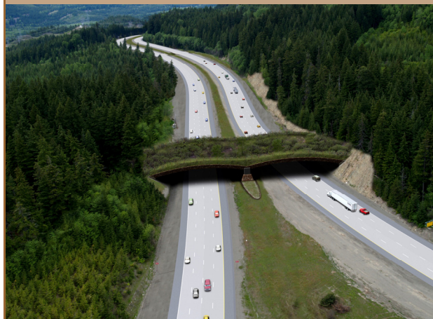
Figure 11: Proposed design of a wildlife crossing near the town of Easton, in the eastern part of the greenway.
