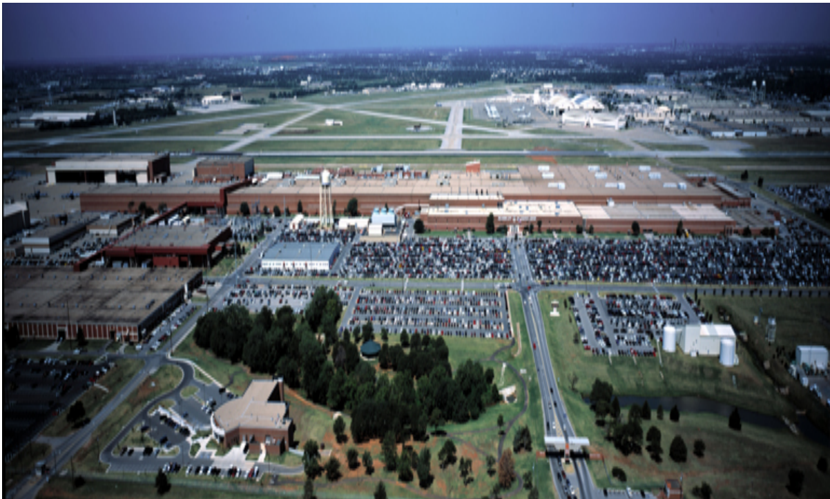
ENHANCED WORKING ENVIRONMENT – Green infrastructure (foreground) east of B-3001 softens the harsh surroundings and provides quality location for a ½ mile fitness trail in the heart of the industrial side of the Base
