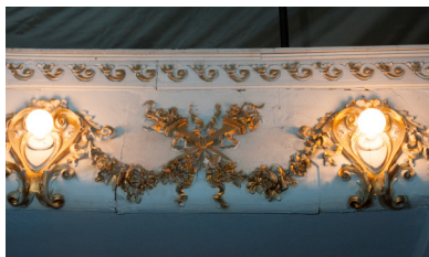
Original architectural details have been retained and restored.
