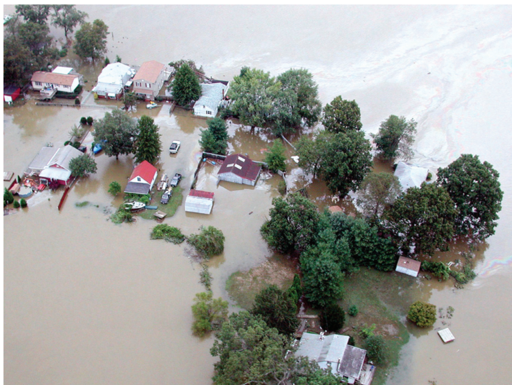
Bayside homes in Bowleys Quarters are surrounded by water the day after Hurricane Isabel. The six-foot storm surge generated by Hurricane Isabel caused extensive damage in this east Baltimore County community.
